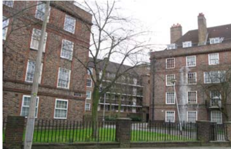
Existing council housing at Clapham Park
