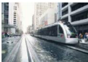
Houston, TX light rail
